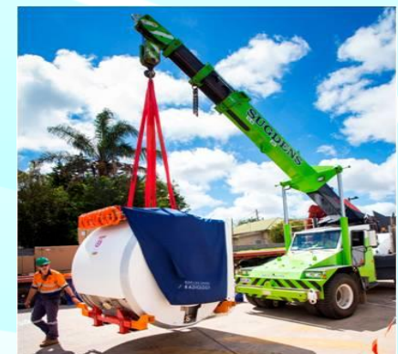
Installation of 3T Wide Bore MRI to Darling Downs Radiology Toowoomba
